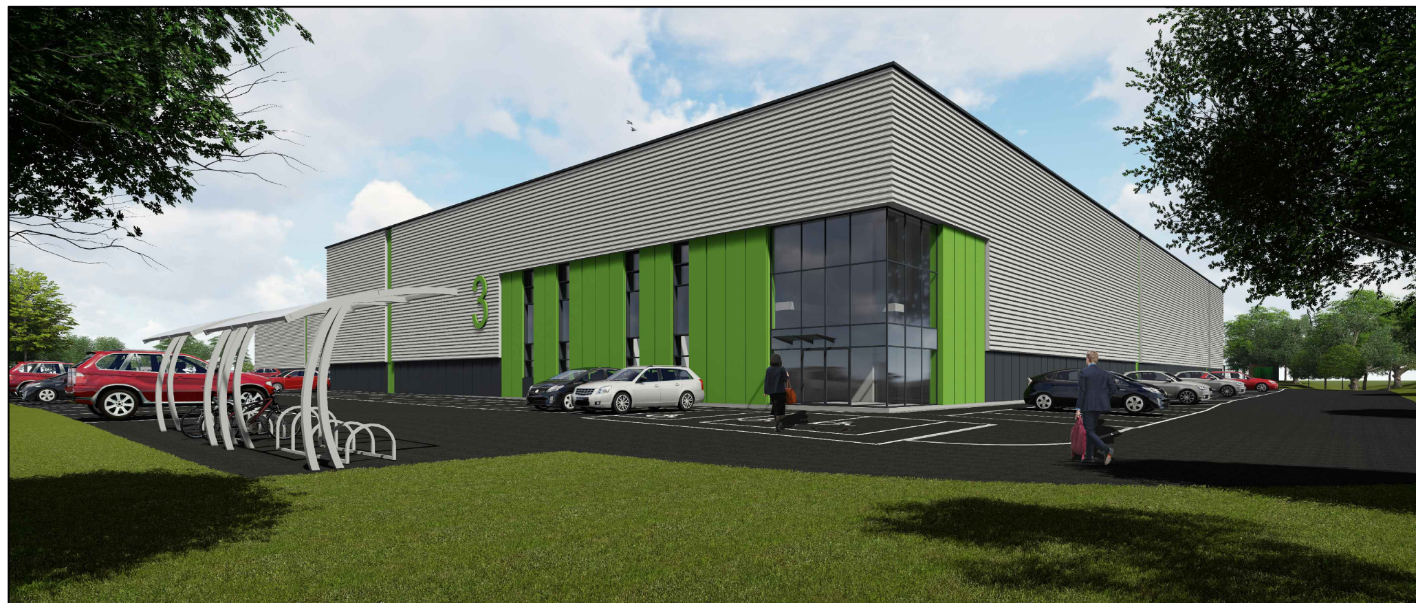
View North East - Unit 3 Office Entrance
